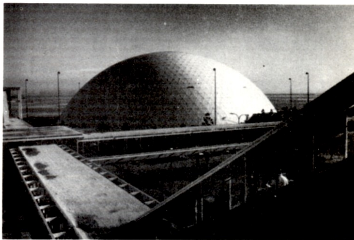
A geodesic dome in Long Beach like the one under construction to house Cinergy.
